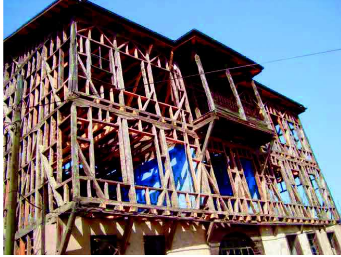
Fig. 10. Establishment of timber frame, Osmaneli
