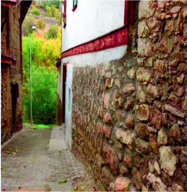
Fig. 2. Foundation Beneath Wall
