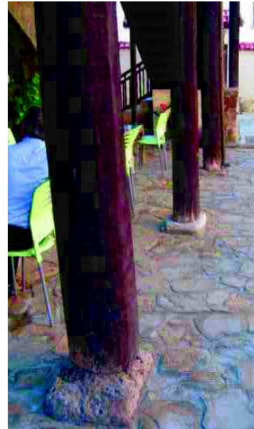
Fig. 3. Independent Stone Foundation
